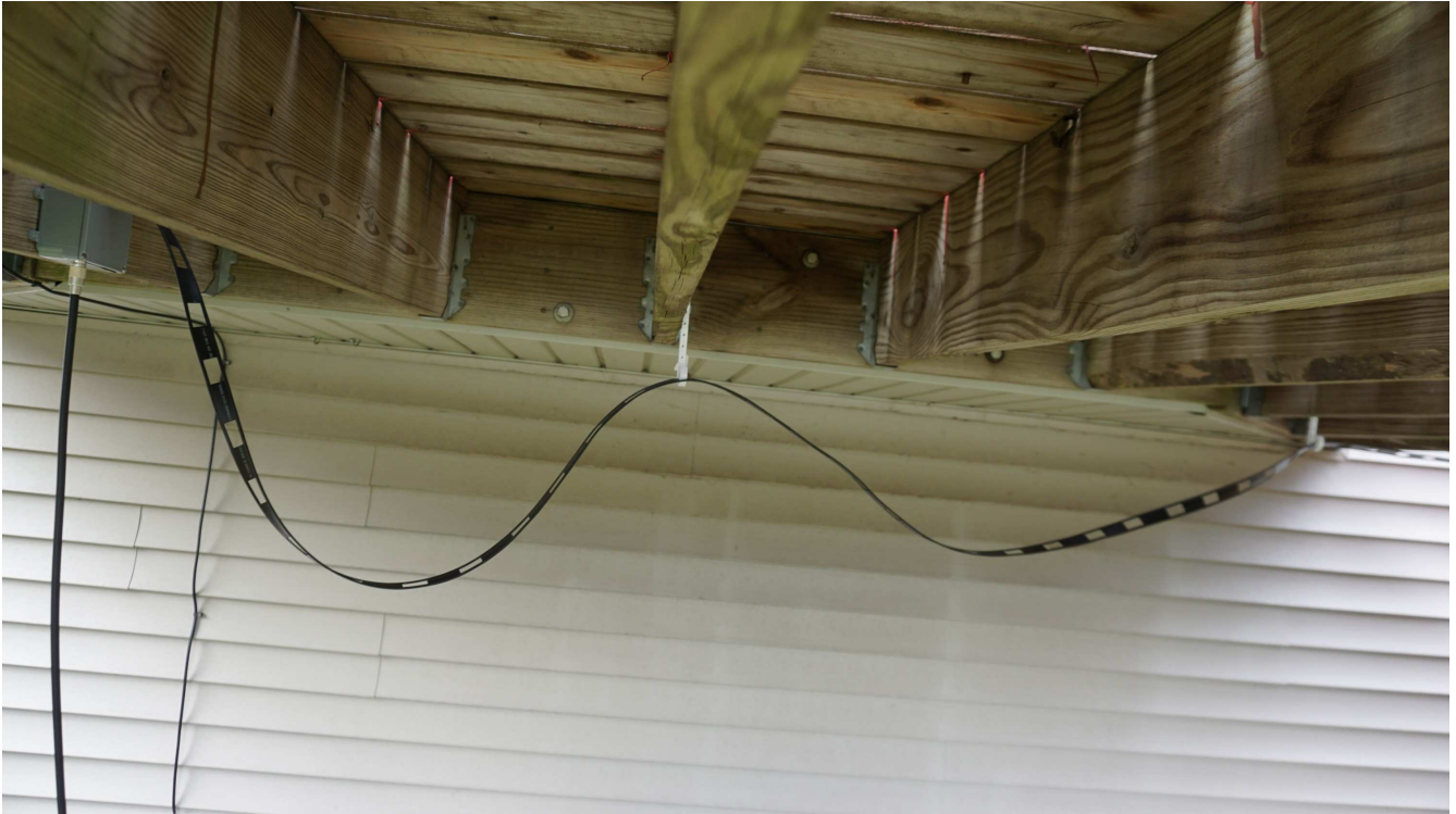
Plastic hanger under deck supporting window line to balun. Hooks are plastic ½" copper pipe hangers available from Lowe's.
