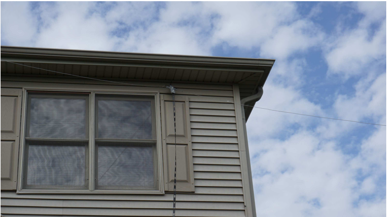
WA1FFL LADDER-LOC mount under eave of house 22 ft above ground level. Right wire goes to bush at 9 feet above ground. Left side goes to tree at 15 feet above ground.
